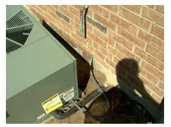
T& P line termination too high. Condensate line for AC unit is buried. See plumbing and AC comments.
